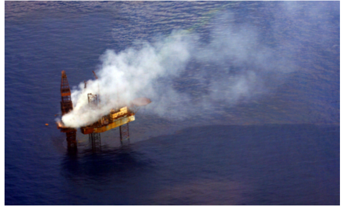
The West Atlas oil rig is still leaking tonnes of oil into the Timor Sea.
